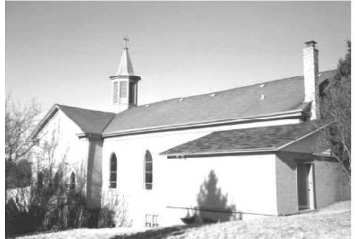
The southwest side of the building as viewed from the rear.
